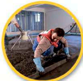
Cement and sand screeds
