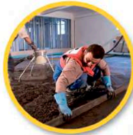
Cement and sand screeds
